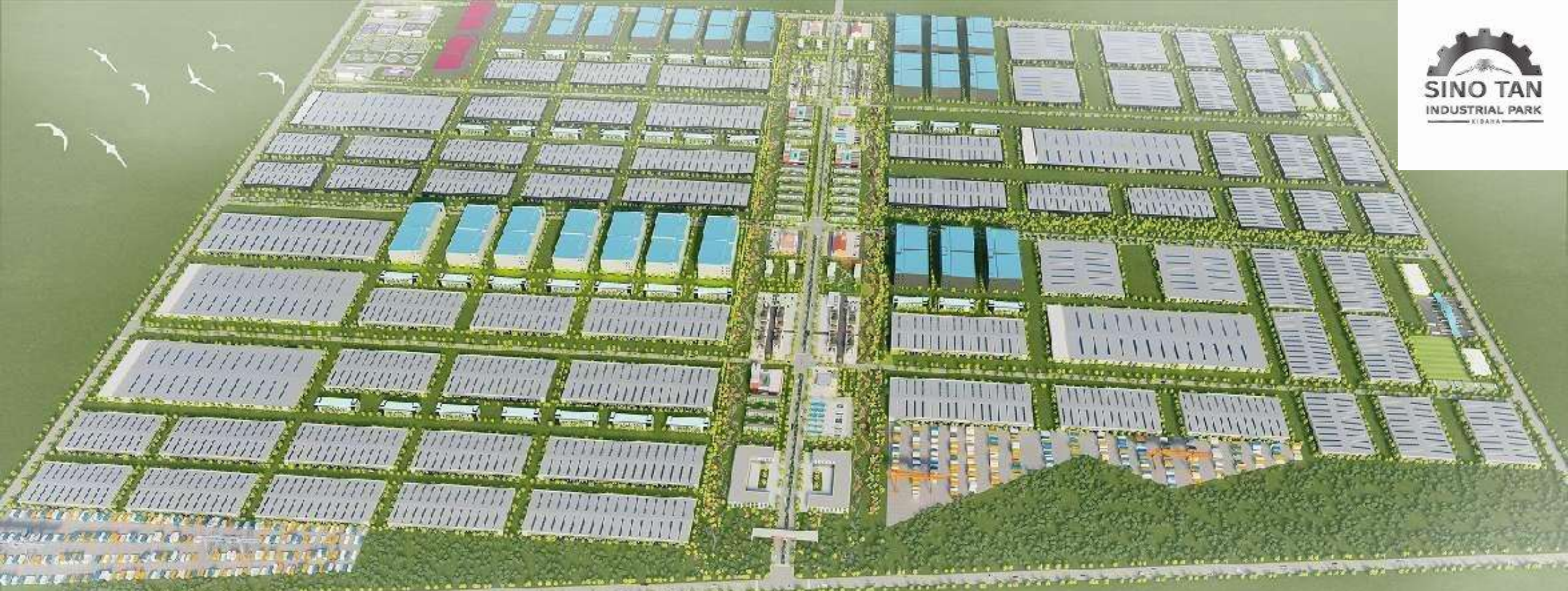
Aerial view of the project
